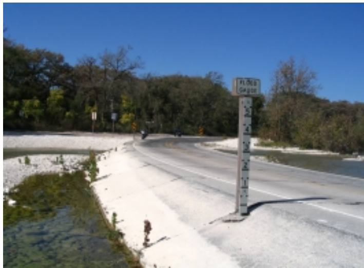
Photo 3 - "Dry" river bed crossing
